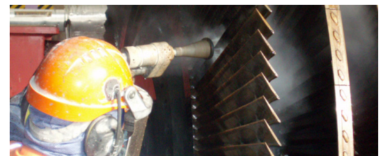
Cleaning deposits from blading
