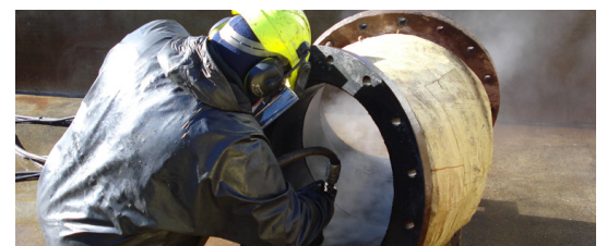
Cleaning paint & corrosion from pipework
