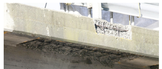
Prepared repair sites
