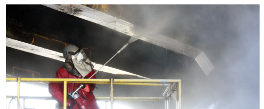
High pressure wash down
