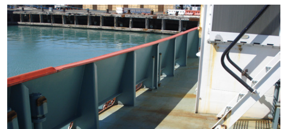
Deck areas before hydroblasting
