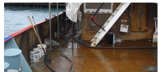
Deck areas after hydroblasting
