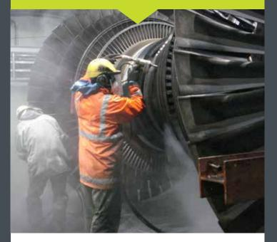
For thermal and geothermal power generation facilities, our unique low-flow rate, but ultra-high pressure pumps allow operators to tackle tight spaces and complex shapes such as cleaning ash from inside boilers or silica scale from turbine blades.
