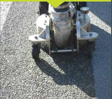
The roading sector in New Zealand has been for many years a significant user of water jetting services for road-line removal and bitumen flushing (also called water cutting) services. Another relevant service is surface preparation prior to applying colourised surfacing e.g. greening.
